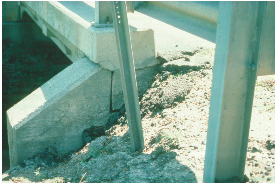
Figure 10.1.52 Roadway Shoulder Erosion Behind Wingwall
