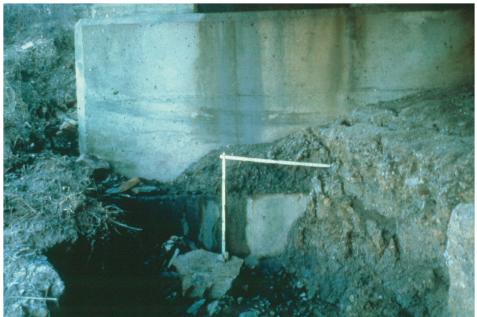
Figure 10.1.28 Erosion at Abutment Exposing Footing
