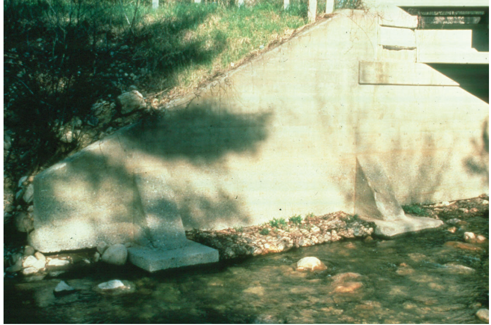
Figure 10.1.51 Scour and Possible Undermining of Concrete Wingwall
