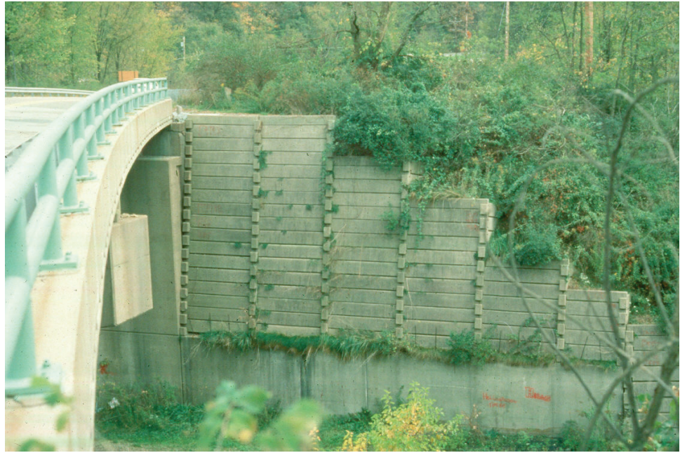
Figure 10.1.42 Straight Wingwall
