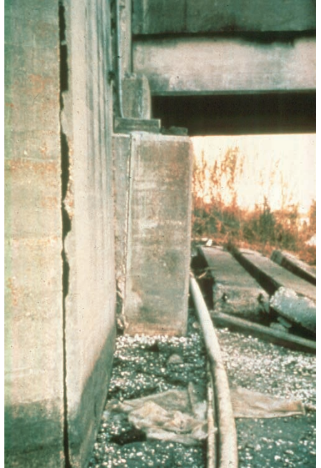
Figure 10.1.30 Rotational Movement at Abutment
