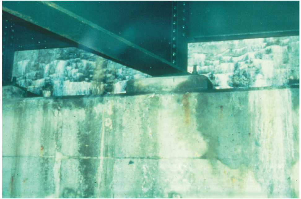
Figure 10.1.33 Deteriorated Concrete in Abutment Backwall
