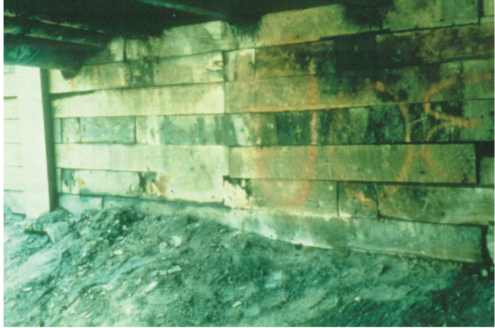
Figure 10.1.37 Decay in Lagging of Timber Crib Abutment
